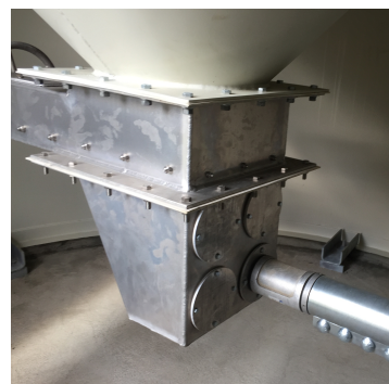
Silo Outlet with Slide Gate and Vacuum Take-off Box
